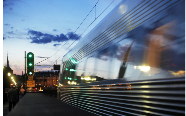
INTERFLO mainline signaling
